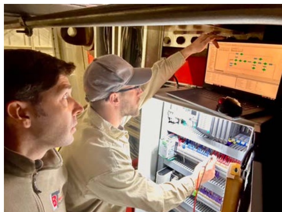
LBTO staff members Alessandro Cavallaro and Dan Rapoza working on the new ASM PLC box inside the telescope central structure. Photo Credit: A. Cavallaro
