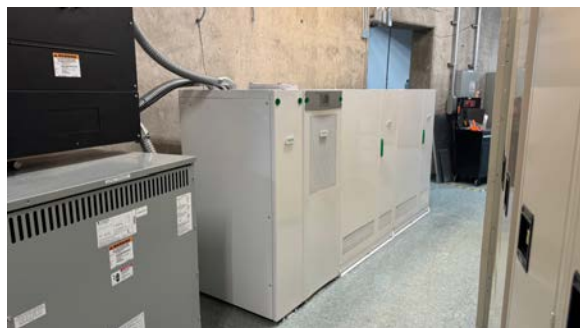
Newly installed Computer Room UPS unit. Photo credit: P. Hartley
